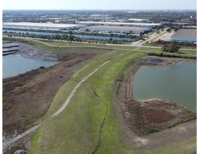
*Figure 4: Previously placed embankment from Railroad Street to Channel Bridge*
