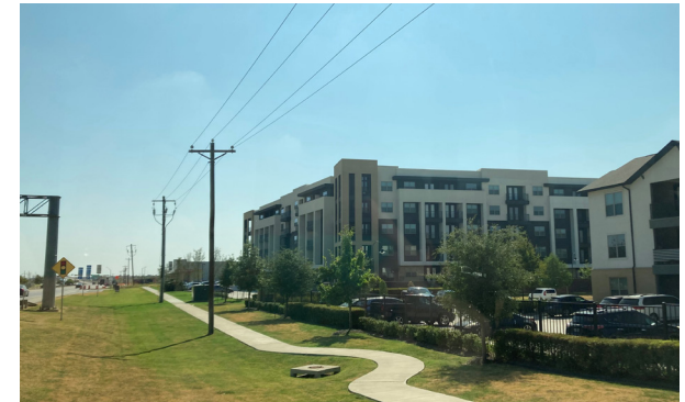
Wide sidewalks were built with the multi-family development.
