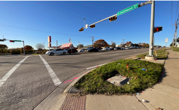
Elements that impact pedestrian safety and comfort include placement of pedestrian signals and alignment of curb ramps.
