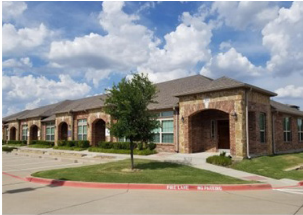
B Vista Ridge Rockbrook Office Park 28,199 SF | 2011-16 YR BLT | $30/SF MG
