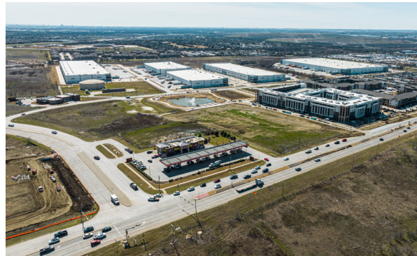
Crown Centre development taking shape near the intersection of FM 544.
