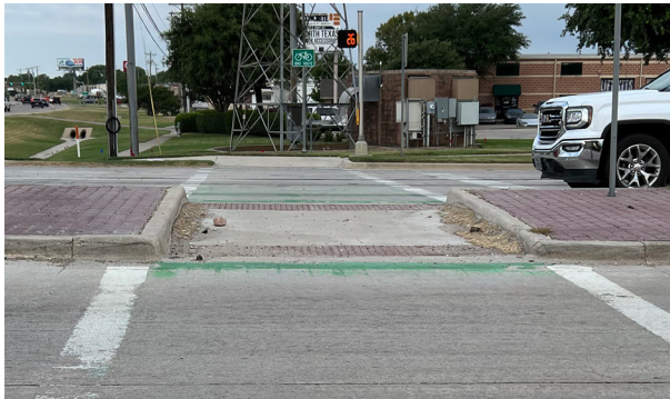
DCTA Trail crossing along Valley Ridge Blvd at Business 121.
