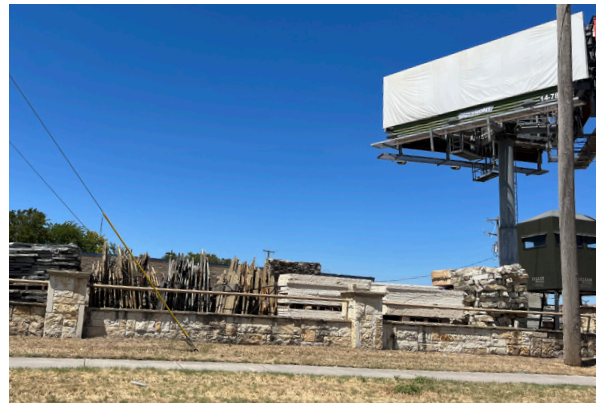
Visible outdoor storage and materials.
