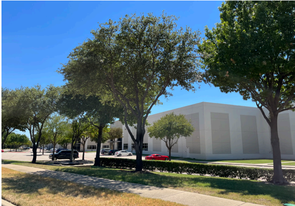
Industrial buildings set away from the roadway.
