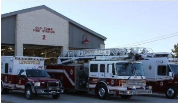
Firehouse #2 is located on Main St just north of the Business 121 Corridor (Source: City of Lewisville).
