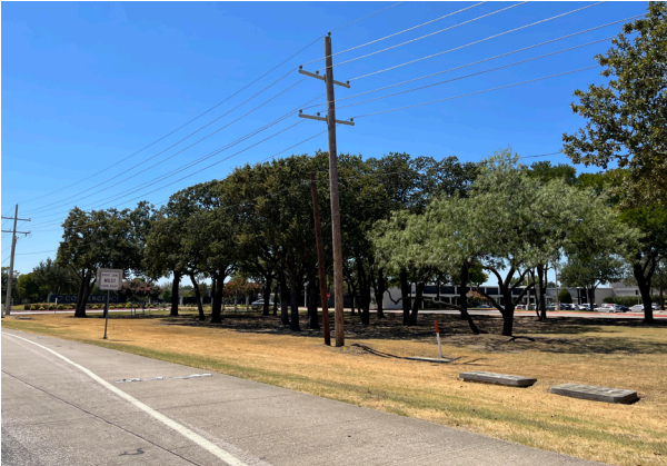
Curbless edge along roadway.
