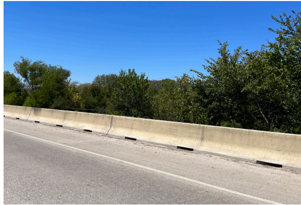
Roadway edge lined with jersey barriers.
