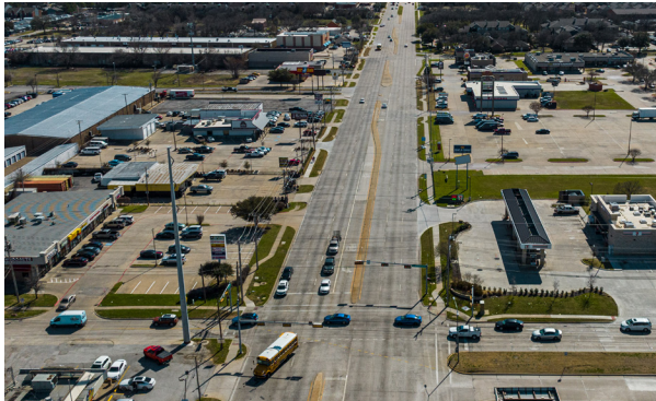
The Corporate Drive area features a high number of driveways; many signalized intersections have a driveway within 250 feet, posing potential safety and traffic flow issues.
