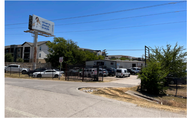
Drainage along the roadway.
