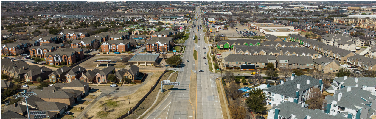
Transition from FM 3040 overpass directly into residential on both sides of corridor.
