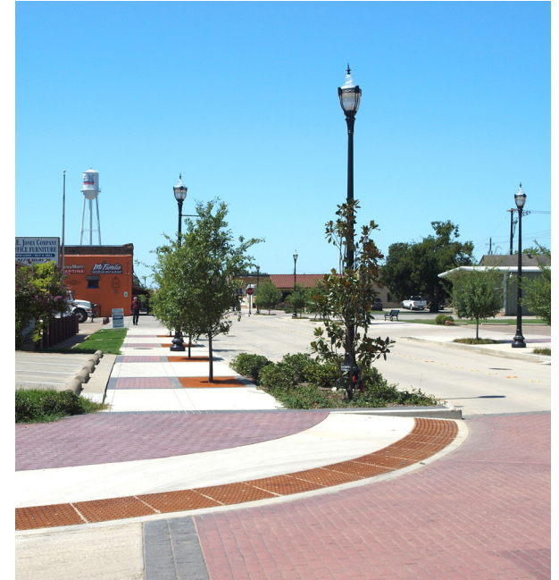
Curb extensions, or bulb-outs, can act as traffic-calming measures by reducing the street width at intersections and the distance pedestrians have to cross.
