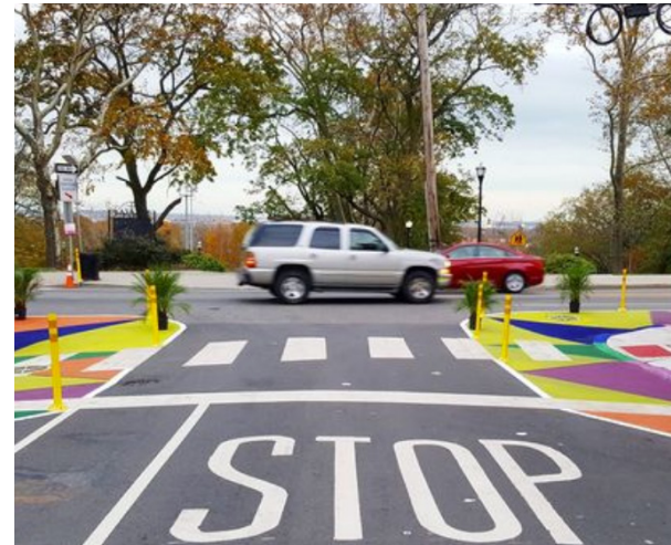
Curb bump-outs and colorful painted crossings can attract attention to - and physically prevent - some collisions.
