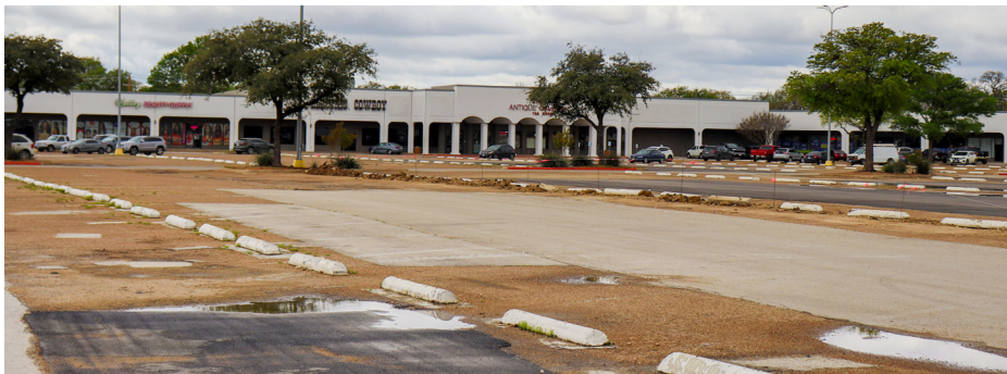
Patch work repairs to the parking lot for the Lakeland Plaza.
