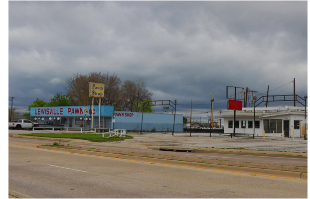
Pawn shop and vacant use on Mill Street in the catalytic site.
