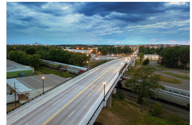
An overpass is used to separate vehicular and pedestrian crossing from rail lines below.
