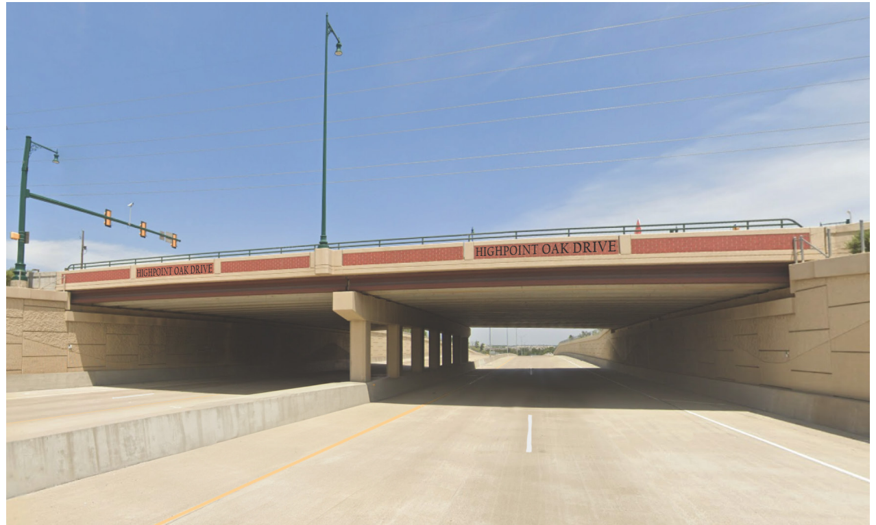
Concept of what the corridor between FM 3040 and the Sam Rayburn Tollway could look like if the main lanes were depressed and the frontage roads kept at grade.
