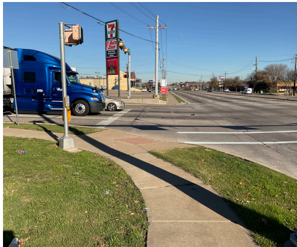
A curb ramp at the Corporate Drive intersection points to the middle of the intersection, posing a safety risk for those in mobility-assisted devices.
